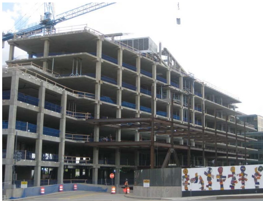
View of the Office Building from M Street Ramp
